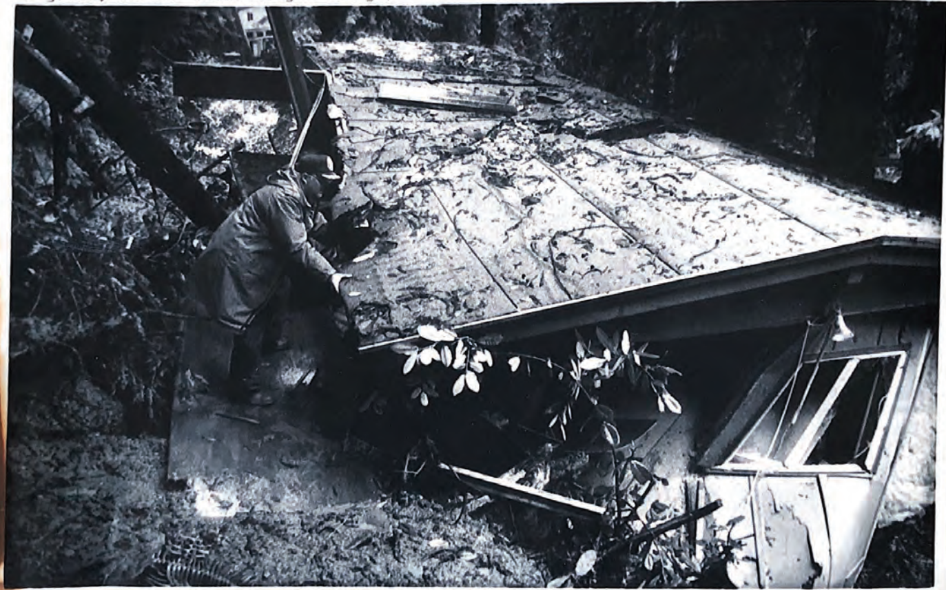
(FX100)BOULDER CREEK, Calif., Feb. 16--SEARCHING FOR OWNER--Rescue worker Leo Kuhnlein of the Boulder Creek Fire Department searches for Amy Ratnofsky, Sunday, who is believed to be buried inside the wreckage of her home. The house was smashed by a mudslide, Saturday, caused by the torrential rains of a severe winter storm. ⊕ (AP Colorphoto)(pbl-11531-Please credit USA Today/Doug Menez) 1986 (EDS: House is green, worker wears bright orange) ⊕
