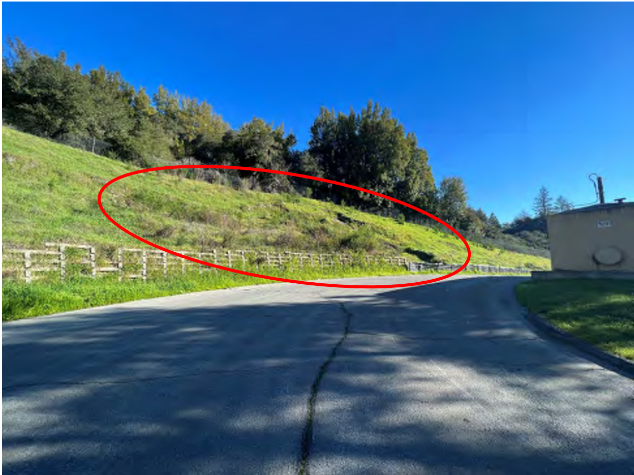
Photo 8. Surficial instability above the access road north of the transfer station building.
