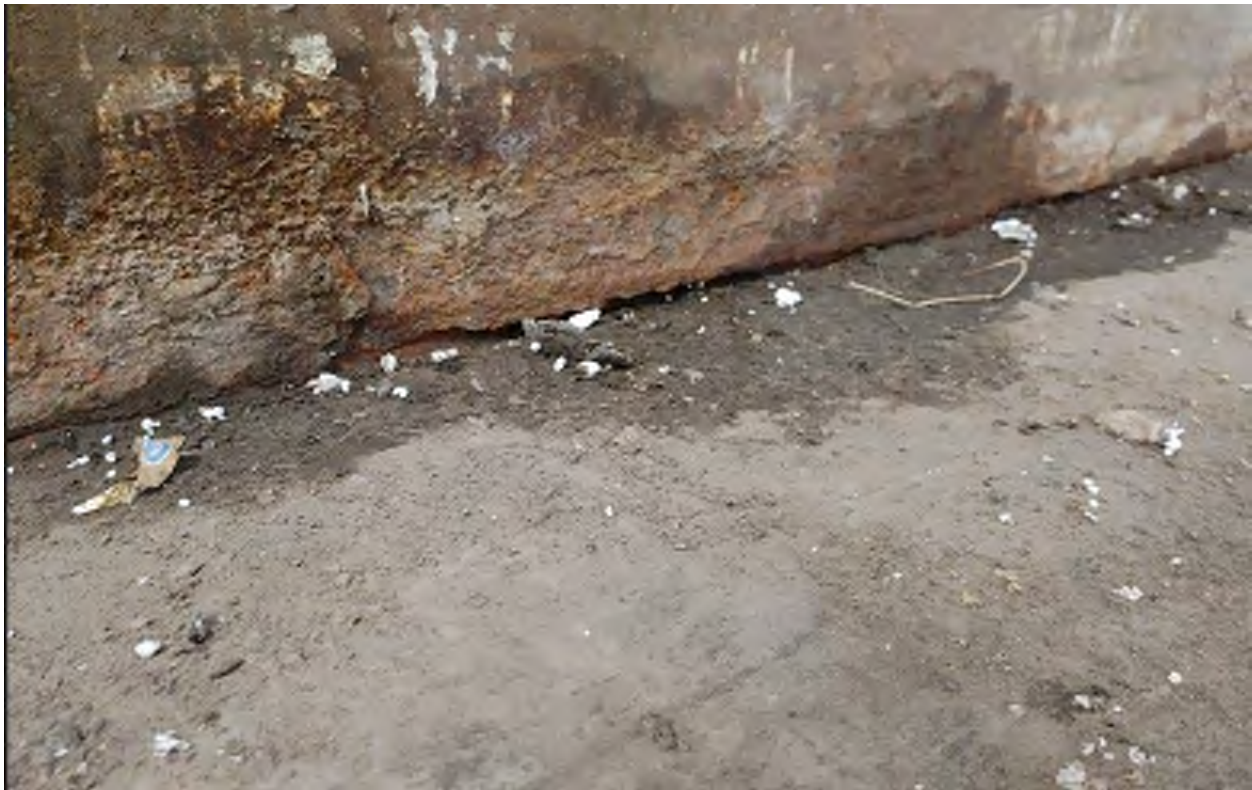
Photo 12. Corroded Protective Steel Plate on the Face of The Retaining Wall
