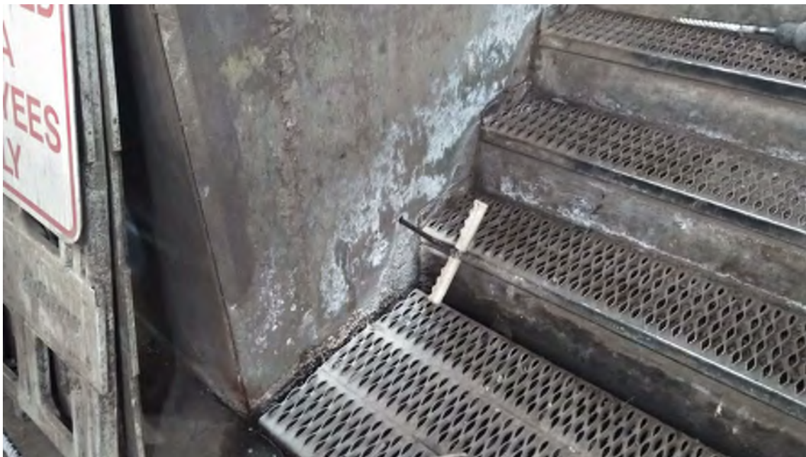
Photo 10. Efflorescence on South Wall.
