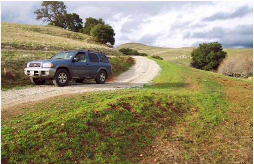
THE SAME ROAD OUTSLOPED WITH ROLLING DIPS
